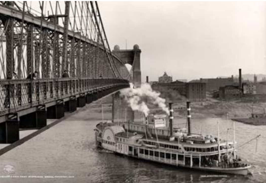
▼ This early twentieth-century photo of Cincinnati (1906) shows The John A. Roebling Suspension Bridge, originally known as the Cincinnati-Covington Bridge. When it opened on December 1, 1866, it was the longest suspension bridge in the world at 1,057 feet (322 meters). This bridge was the test model for Roebling's more famous 1883 design – The Brooklyn Bridge in New York City.
