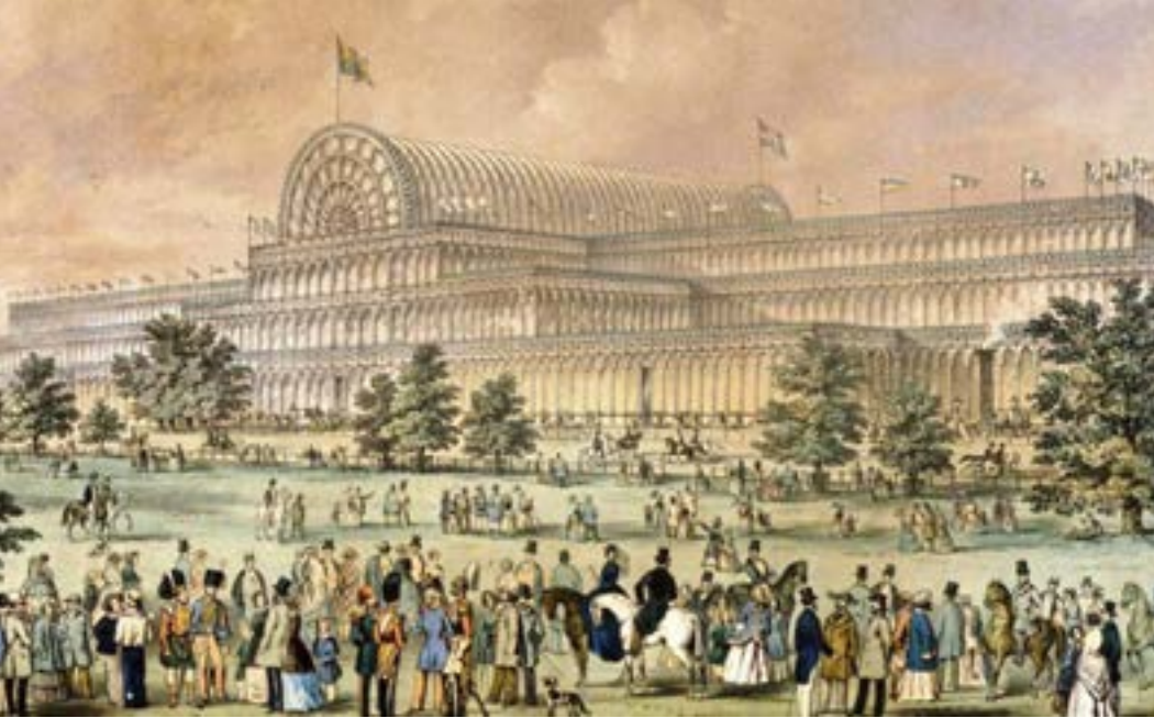
▲ Crystal Palace, the giant glass and iron exhibition hall that housed the Great Exhibition of 1851 in Hyde Park, London. Designed by Sir Joseph Paxton, it consisted of an intricate network of slender iron rods sustaining walls of clear glass. On the ground floor housed more than eight miles (thirteen kilometers) of display tables, showcasing over 14,000 exhibitors.
