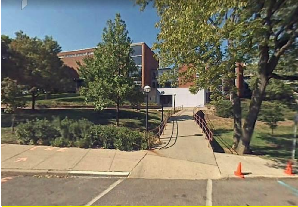
Blue Box Entrance on Clifton Court
